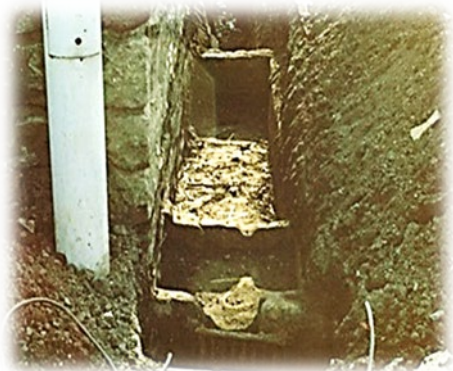
Two chamber horse trough, revealed during 1989 drain repairs: Photo John Lambert.
